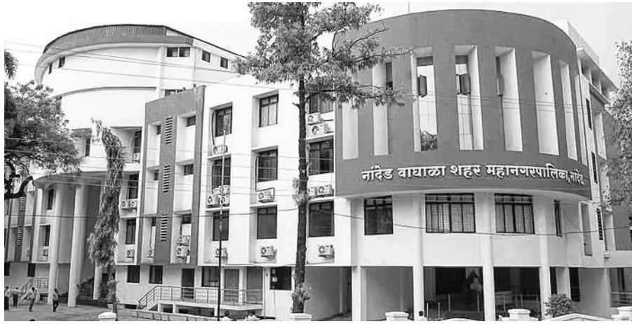
There are 64,858 legal water connections in the jurisdiction of the NWCMC and many illegal connections
