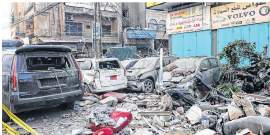
A residential building whose top two floors were hit by an Israeli strike in the Ghoberi area of Beirut's southern suburbs. -AFP
