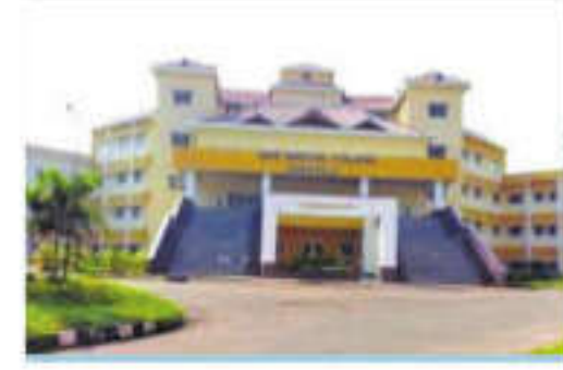
Overgrown grass and bushes have taken over the premises of the building and students and staff members are afraid to go near it. The situation is worsening — A source at Paripally Medical College
